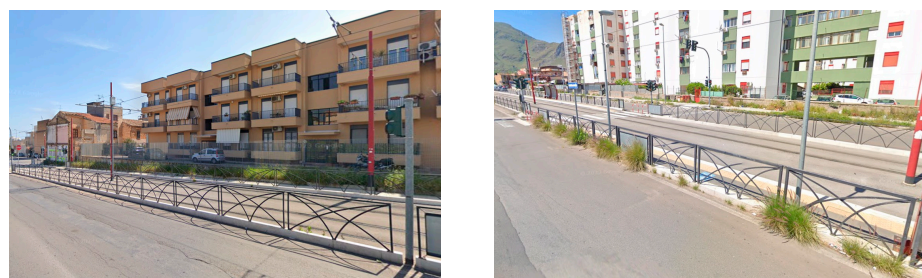
Figure 23. Photos of the analysed road pavement (via Antonio Laudicina)—class E tramway line.
