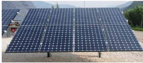
Figure 5.10: The analysed PV systems at ABD: mono-crystalline back-contact technology [source:Eurac].
