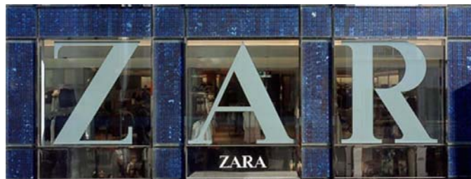
Figure 2.7: warm façade solution. Zara Fashion Store, Cologne, Germany, Architekturbüro Angela und Georg Feinhals: opaque monocrystalline cells combined with transparent glazing in post-beam curtain wall structure, © Solon.
