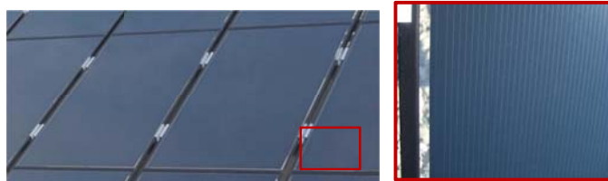
Figure 3.29: Visibility: module aesthetical perception vs observer position. The first picture is taken at a distance of 3 meters and the modules surface appears as an homogeneous pattern; the other picture is taken at a distance of 50 cm: the pattern appears marked by vertical lines, which are the cell connections
