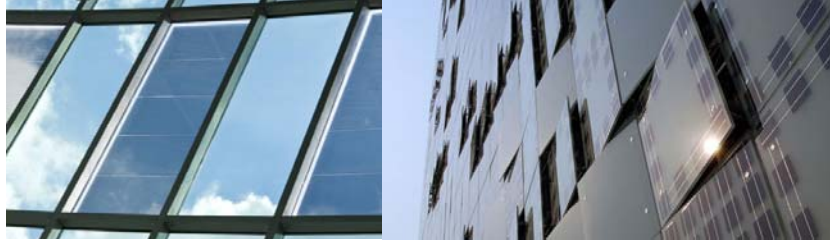
Figure 2.8: Left: Schott Headquarter Mainz, translucent thin film module, © Schott; right: GreenPix Media Wall, Beijing, China, Simone Giostra & Partners, frameless modules with spider glazing system, © Simone Giostra & Partners/Arup.
