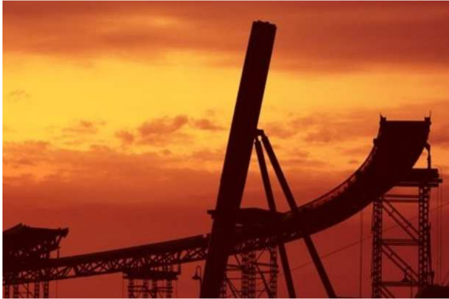
Figure 5.7: Progress of the construction work in site.
