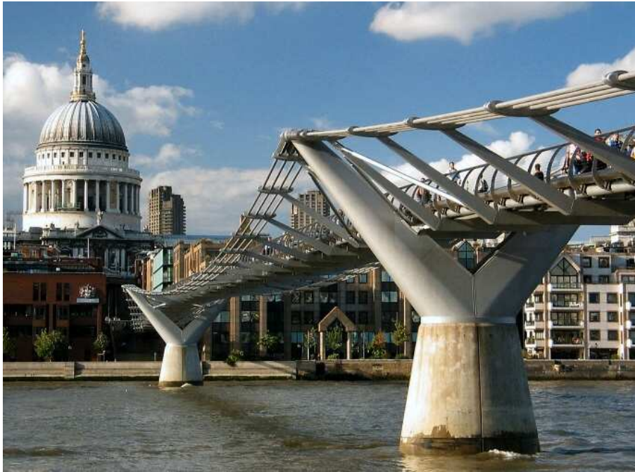
Figure 2.3: London Millenium Bridge
