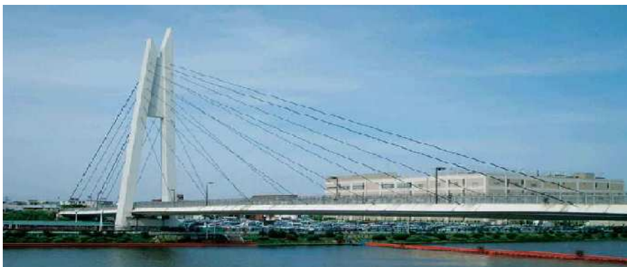
Figure 2.4: Toda Park Bridge, Japan
