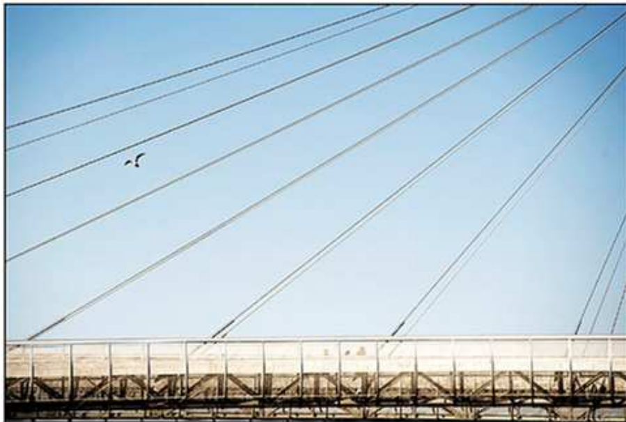
Figure 5.15: Arrangements of the cables after final construction
