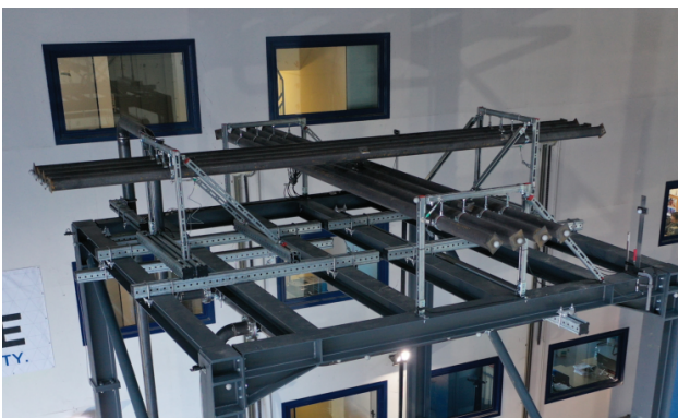
Figure 7: Pipe rack on the third floor
