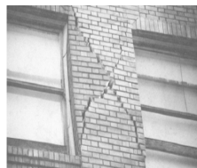
Fig. 2. Diagonal cracks.
