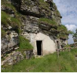
Trenches Sasso Gordona State of abandonment
