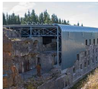
Fort Campo Lusern Recovery with care
