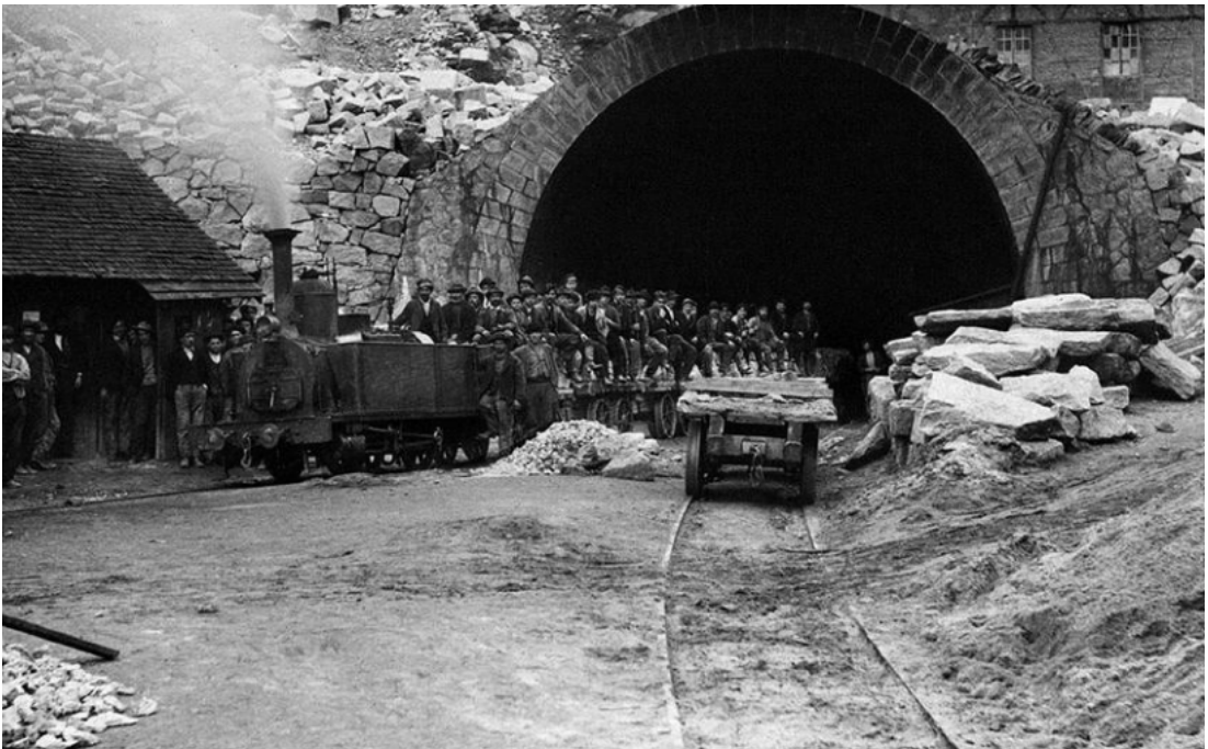
Pic. 2.8 - Workers in front of the north portal of the tunnel under construction (Gotthard). Detail of an Adolphe Braun photograph, ca. 1880.
