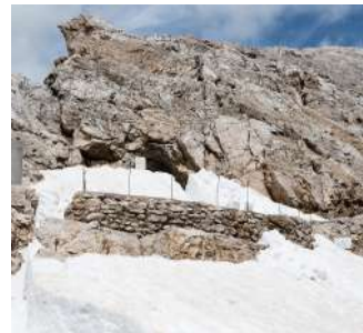
Marmolada Fortifications Recovery with care
