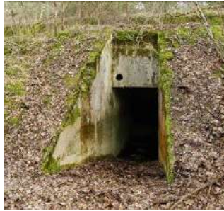
Ouvrage de Ropage State of abandonment
