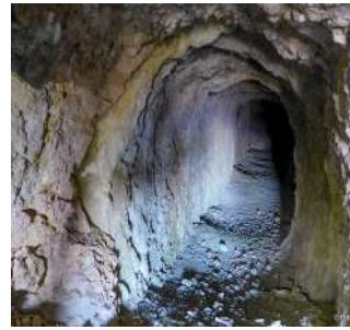
Rock tunnels Monte Calisio State of abandonment
