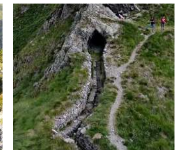
Brembana Valley Trenches State of abandonment
