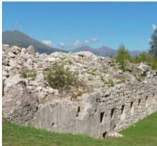
Fort Pozzi Alti Recovery with care
