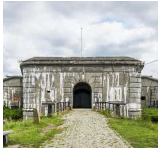
Fort Kessel - Antwerp Recovery with care
