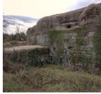
Fort Vrmac State of abandonment
