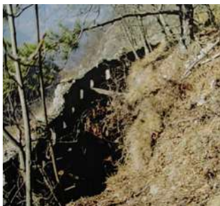
Monte Bondone fortifications State of abandonment
