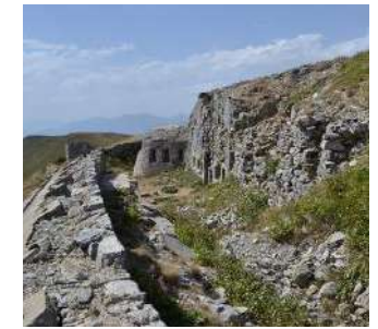
de La Forca Fort State of abandonment
