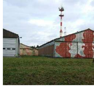
Fort de Machovelette - Namur High level of transformation
