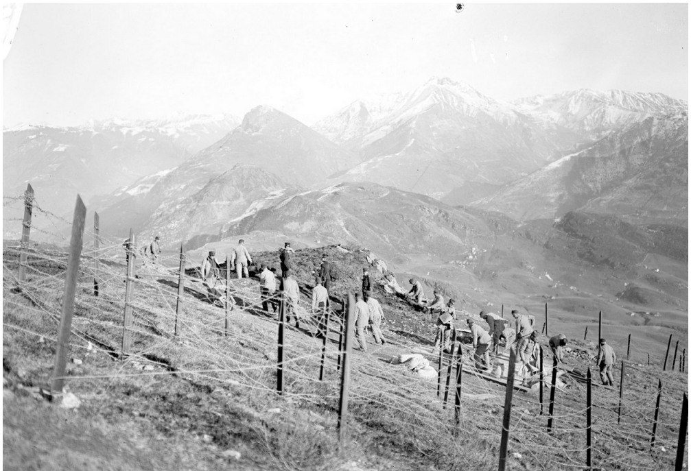
Entrenched systems - Monte Ceneri Wartime
