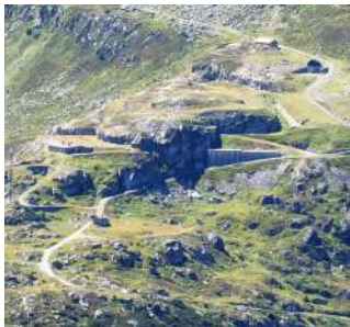
Fort Bazberg State of abandonment
