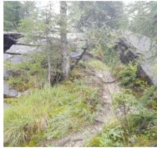
Fort Heideck State of abandonment
