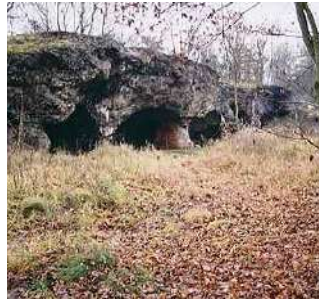
Fort Lasek Destruction - loss
