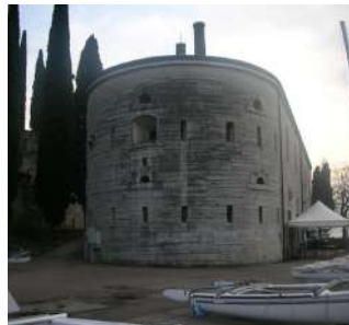
Fort S.Nicolò Recovery
