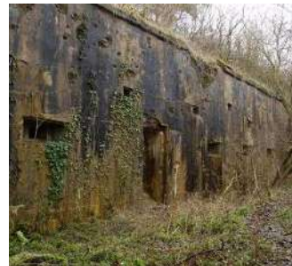
Fort Vaucherauville State of abandonment
