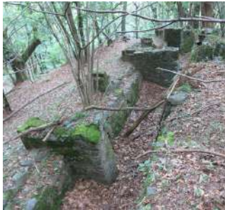
Trenches Magadino State of abandonment
