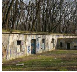
Krakow - Fort 48 State of abandonment
