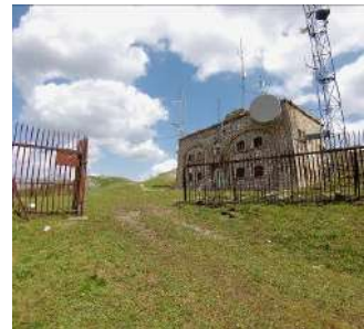
Fort Gondran High level of transformation
