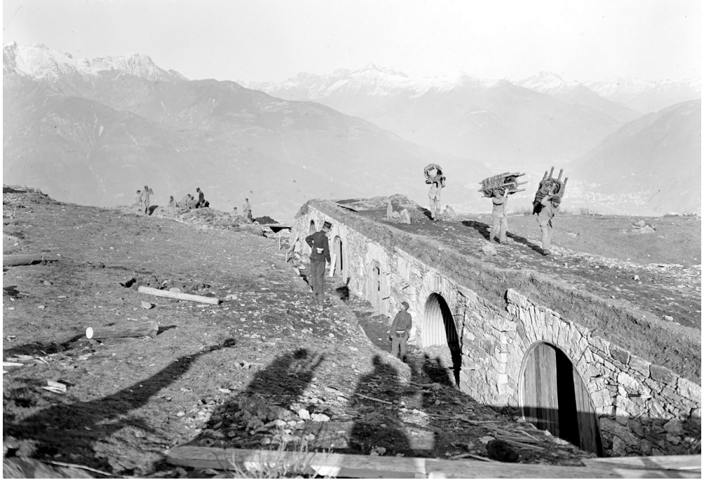
Entrenched systems - Monte Ceneri Wartime
