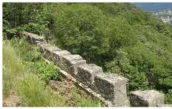
Trenches, Nago (TN) - Italy
