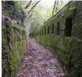
Trenches Monte Orsa State of abandonment
