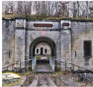
Landrecourt Fort State of abandonment
