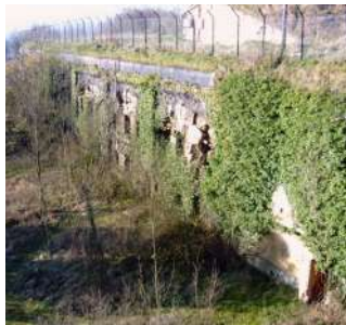
Fort Diou State of abandonment
