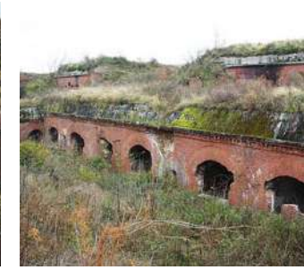
Fort v State of abandonment
