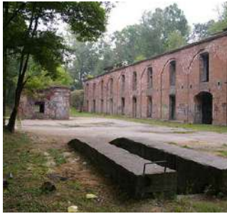
Krakow - Fort 52 State of abandonment
