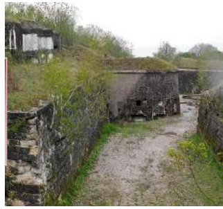
Sartelles Fort State of abandonment
