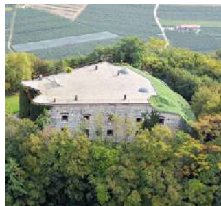
Romagnano Fort Recovery
