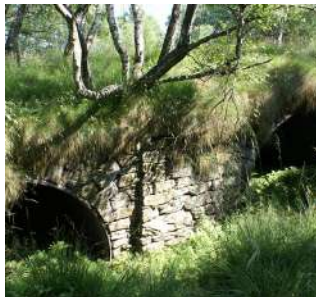
Fortification Monte Ceneri State of abandonment
