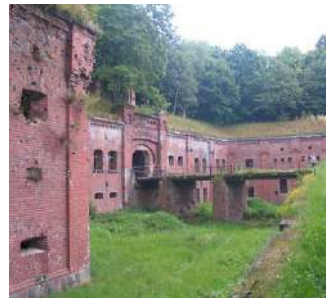
Fort Va - Konigsberg High level of transformation
