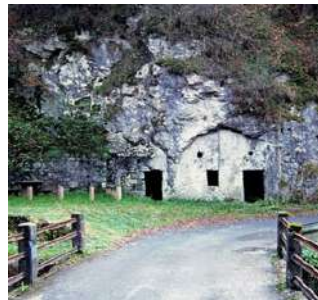
Fort Revegler Destruction - loss
