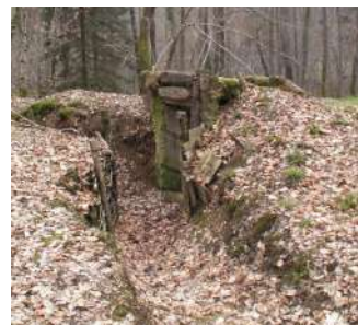
Trenches - La Largue State of abandonment
