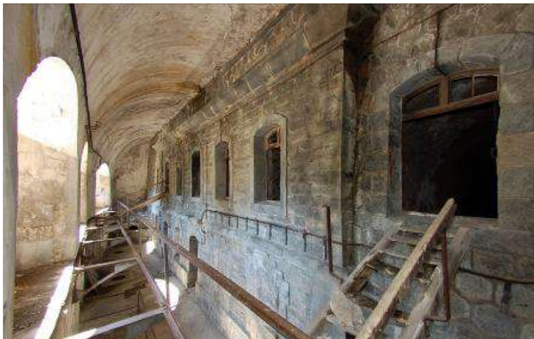
Pic. 2.37 - Reinforcement of existing forts after 1885 using reinforced concrete.
