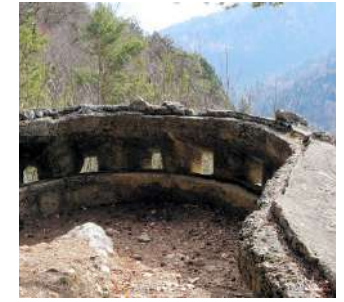
Entrenched system Monte Celva State of abandonment
