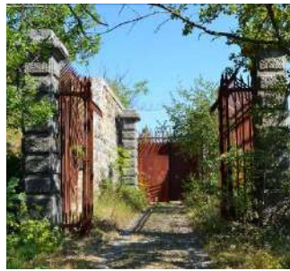
Picciarvet Fort State of abandonment
