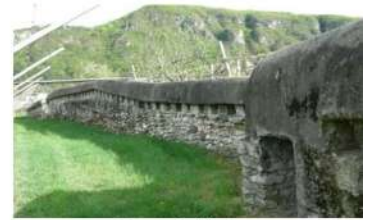
Covered rifle room Marani di Ala (Vallagarina - TN) - Italy
