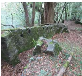
Trenches Magadino State of abandonment
