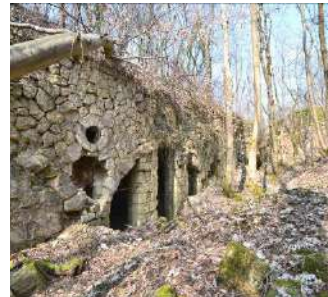
Fort Tannes State of abandonment
