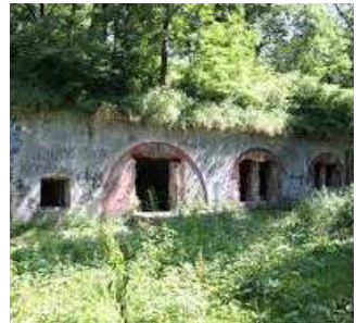
Krakow - Fort 14 State of abandonment
