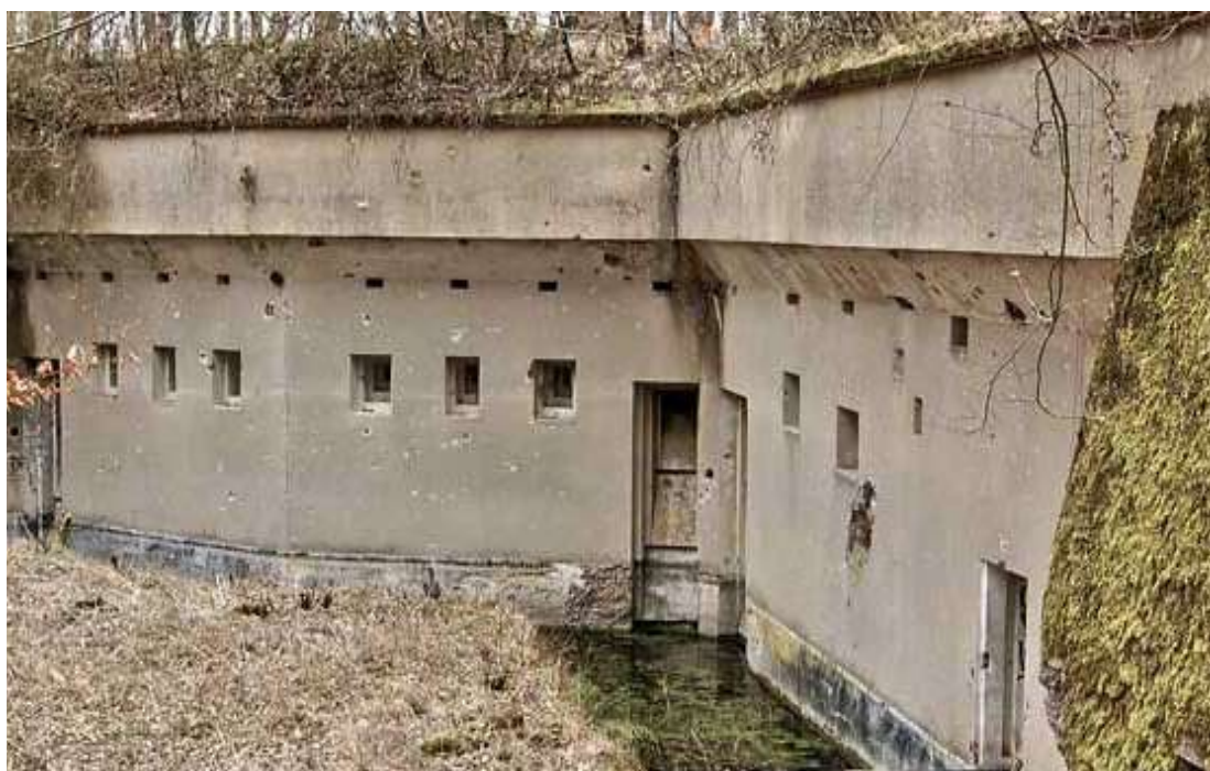
Pic. 2.38 - Reinforcement of existing forts after 1885 using reinforced concrete.
