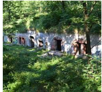
Krakow - Fort 50 State of abandonment
