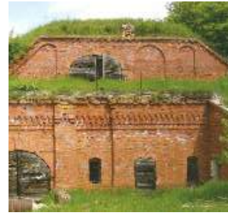
Fort V State of abandonment
