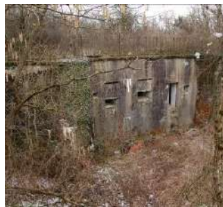
Dugny Fort State of abandonment
