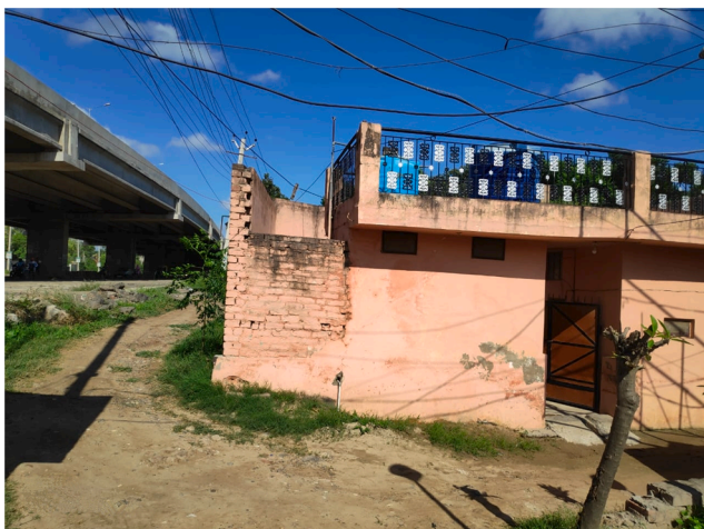
Fig. 3. The highway looming over the mutilated house and the new wall
