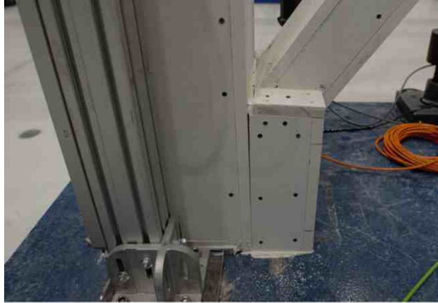
Figure 8.56: Damages after two seismic tests at 1.0g
