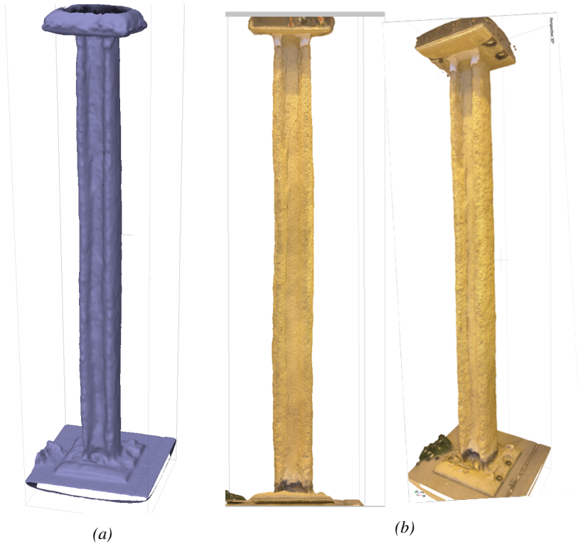
Figure 6.67: 3D model of the column #D obtained using the photogrammetry methodology: a) wired model; b) Textured model.
