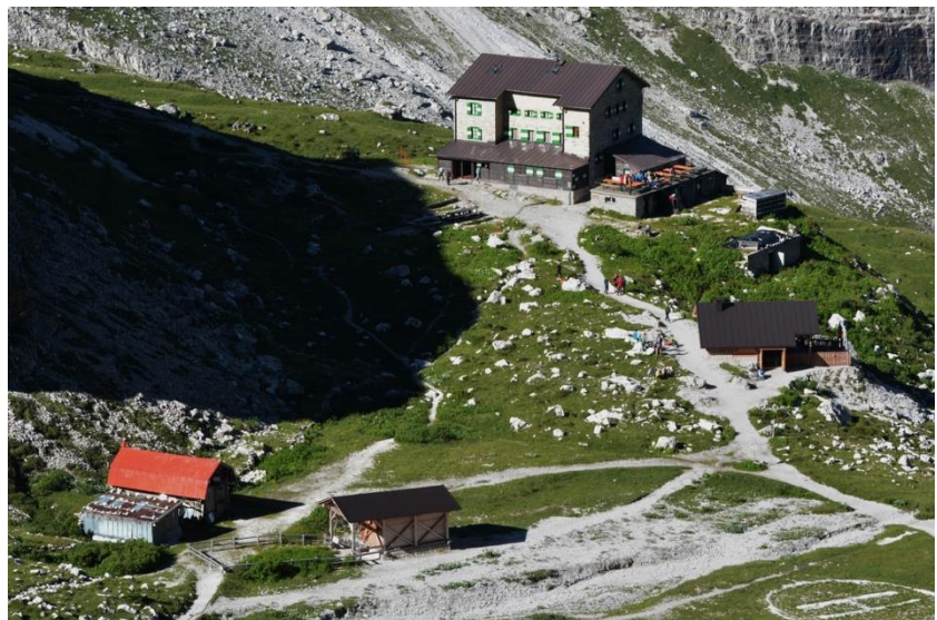
Figure 106. Existing condition of Brentei refuge location
