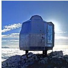
Fig. 122. Bivouac Bruno Ferrario, Grignetta (Lecco), 2178 m a.s.l., 1968, central layout, top porthole, geodetic volume
