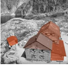
Figure 94. Italian approach: additions to the original “cubo” building in the Refuge Ottone Brentari at Cima d’Asta
