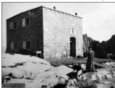
Fig. 79. Refuge Ottone Brentari, Cima d'Asta, 1908, an example of Cubo SAT building type.
