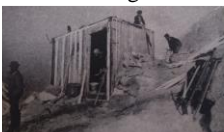
Fig. 75. Refuge au Col du Midi, Guides Courmayer, 1863. In the picture restructuring of 1895.
