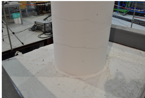
FIG. 5.91 After test 30 cm column 120%
