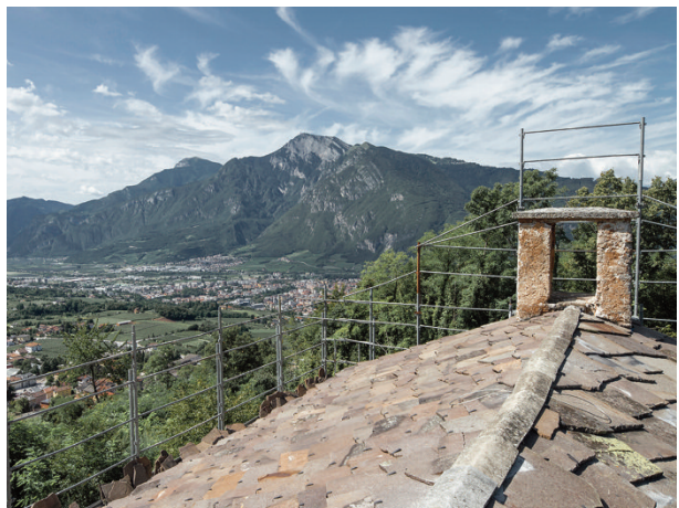
Fig. 10 | St. Agatha Church with the new roof (credit: F. Giampiccolo, 2019).
