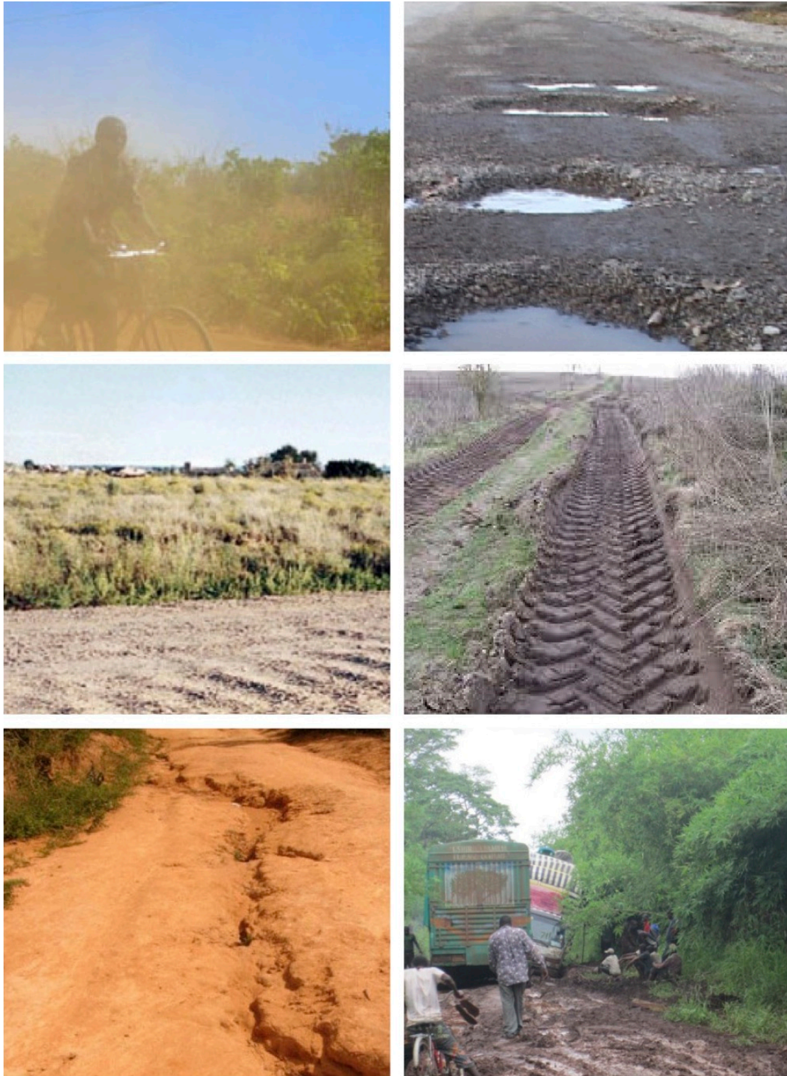
Figure 11 Most common defects associated with dirt roads in Southern Africa.
