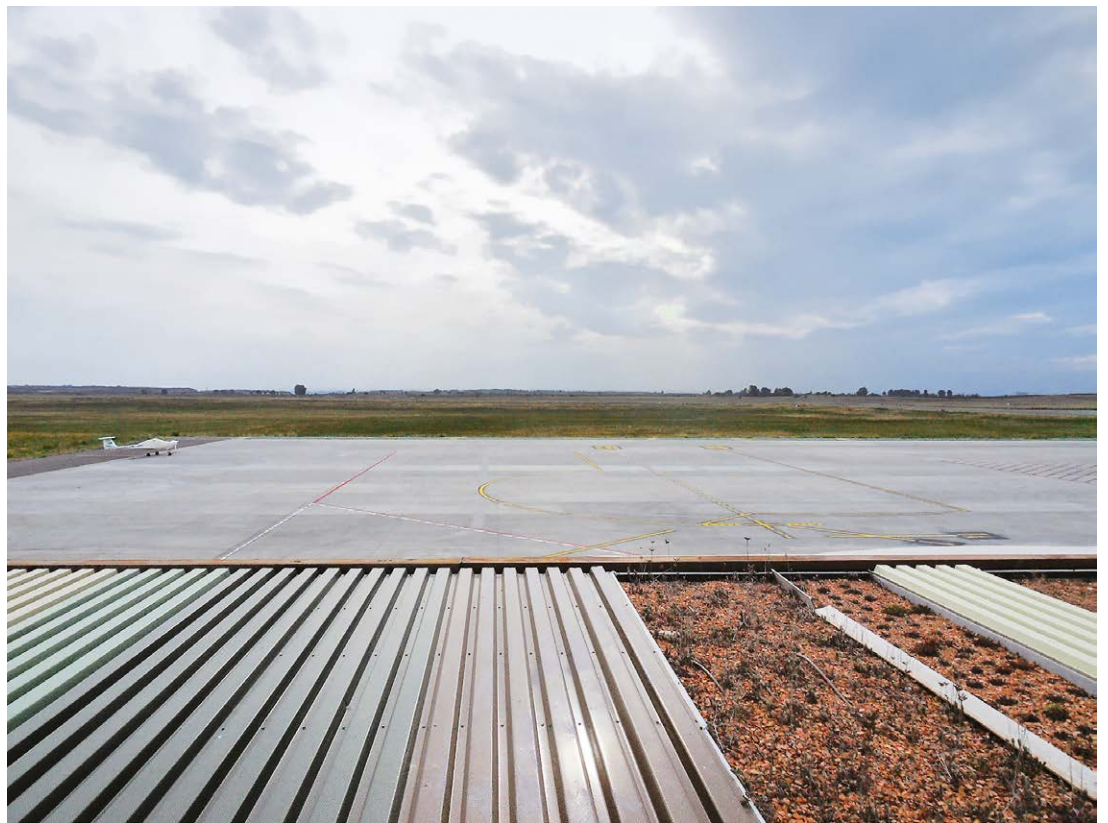
Figure 14 The main envelope is conceived as a continuous blanket covering the most visible faces of the building to give formal unity to the whole and consolidate its presence into the context. The cover has vegetal layers combined with strips of wood and veneer that emulate the vegetable-farming plot environment, and also act as a thermal barrier.
