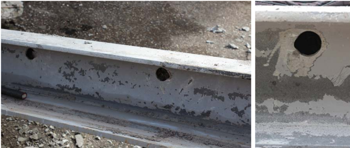
(d) deformations in the holes of the steel web after completion of the tests
