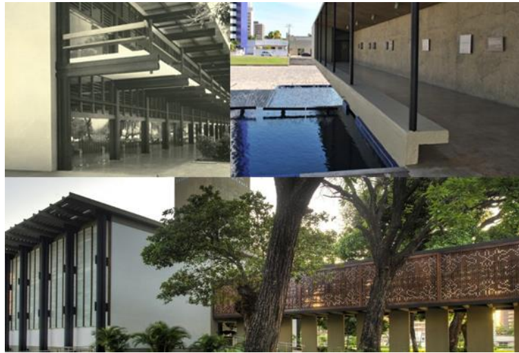
Figure 3 Varandas and overhangs at the Governor's Palace 6 ; Mausoleum – intermediate covered area that connects inside and outside 7 ; Elevated walkway after the intervention 8
