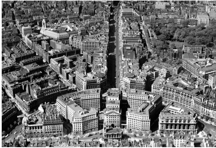
Figure 3. Kingsway aerial, (1946). http://www.britainfromabove.org.uk/image/eaw000649
