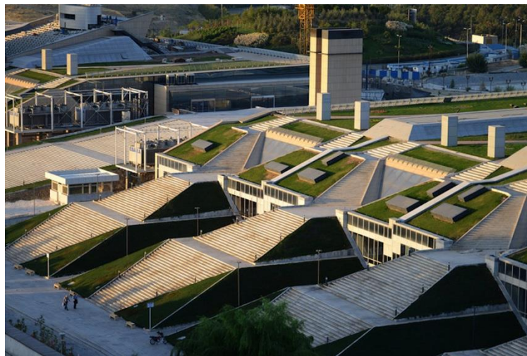
Figure 3. Green roof of Tehran book mall
