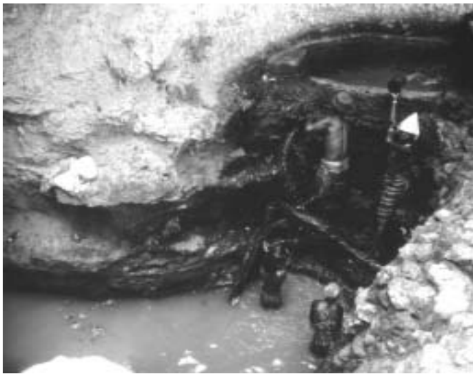
Figure 3. Borana tulaa well. Between the trough and the well shaft there are intermediary reservoirs. Water is lifted rapidly by flinging small buckets (traditionally made of giraffe-hide) from hand to hand. Outside the narrow shaft the speed of water extraction may reach 340 litres per minute. (Courtesy Marco Bassi)
