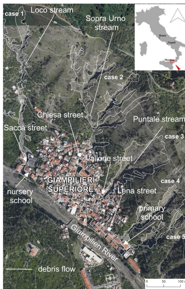
Fig. 1 October 2009 debris flows occurred in Giampileri
