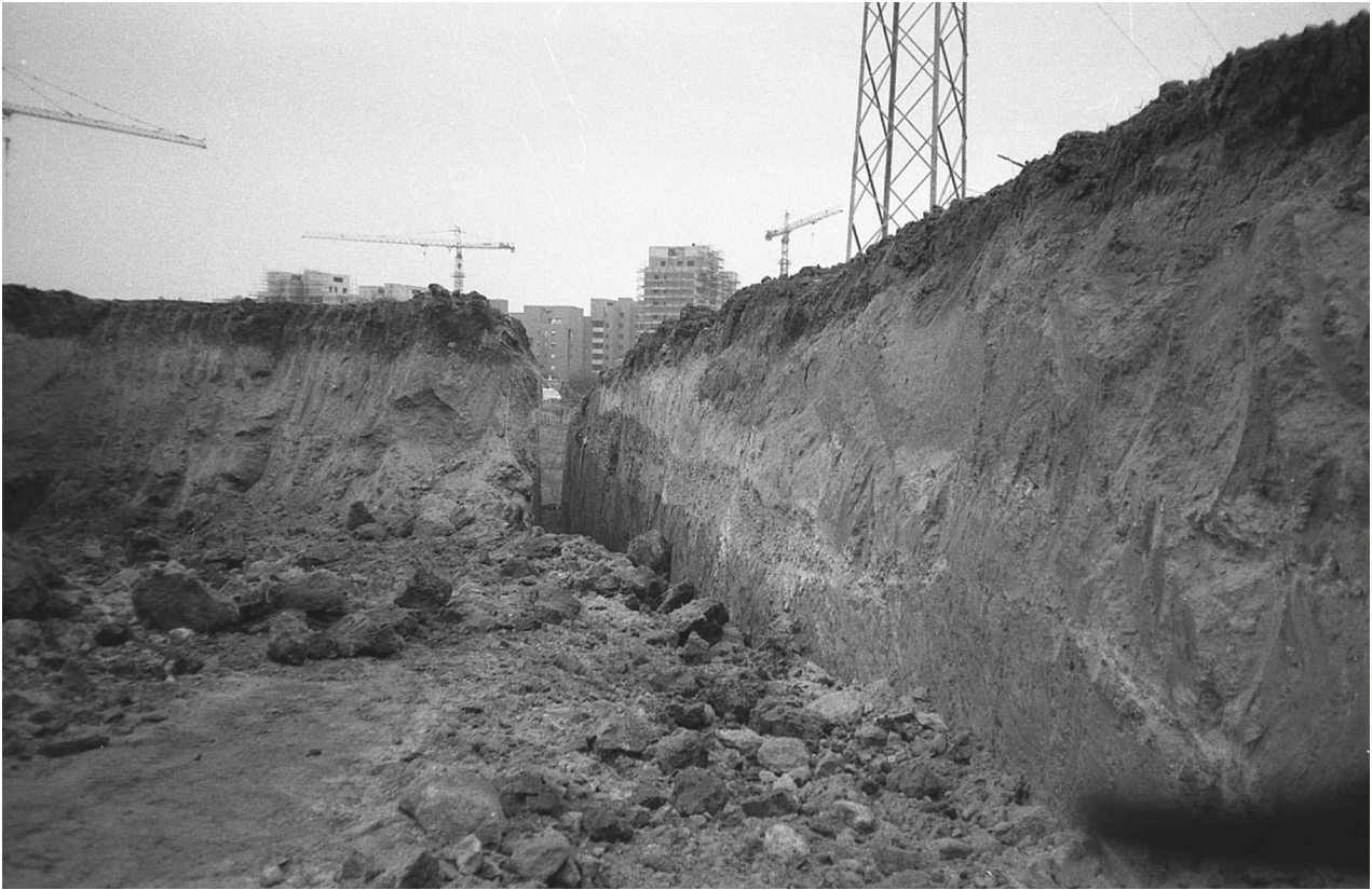
Fig. 14 - Detail of the excavation area showing the fluvial deposits where the archeological site was identified.
