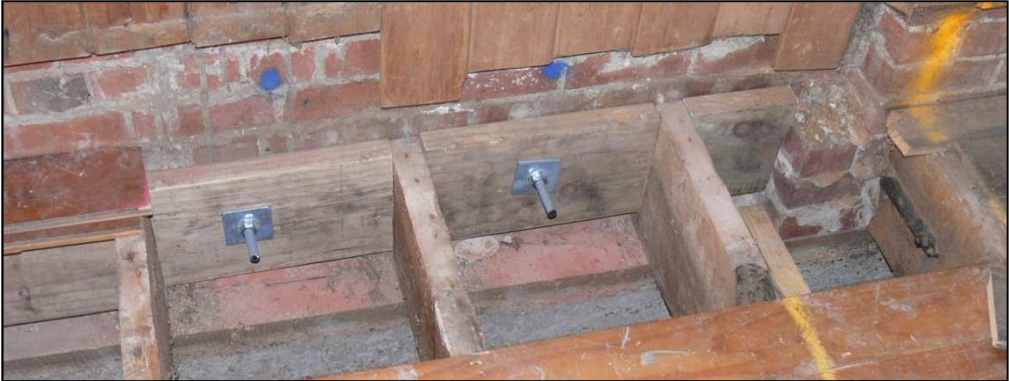
Fig. 5.5 Installation of the new anchors.
