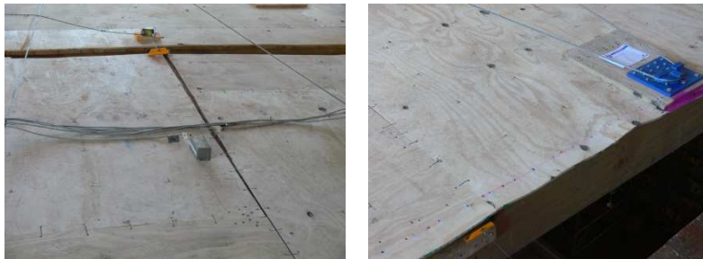
Fig. 5.23 Test 43_C a) panel gap widening b) plywood buckling
