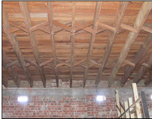
Fig. 5.2 Cross bracings.
