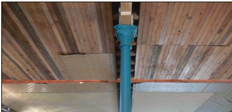
Fig. 5.3 Ceiling boards and metal sheathing.
