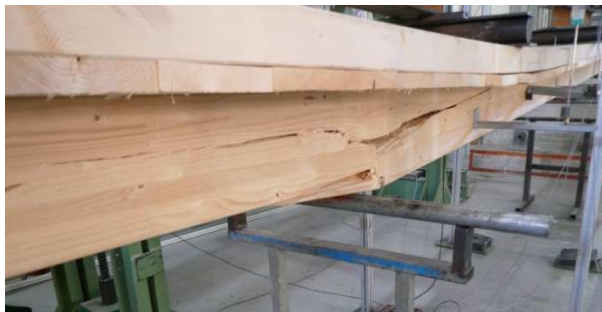
Fig. 6.5 Floor 1 – collapse mode
