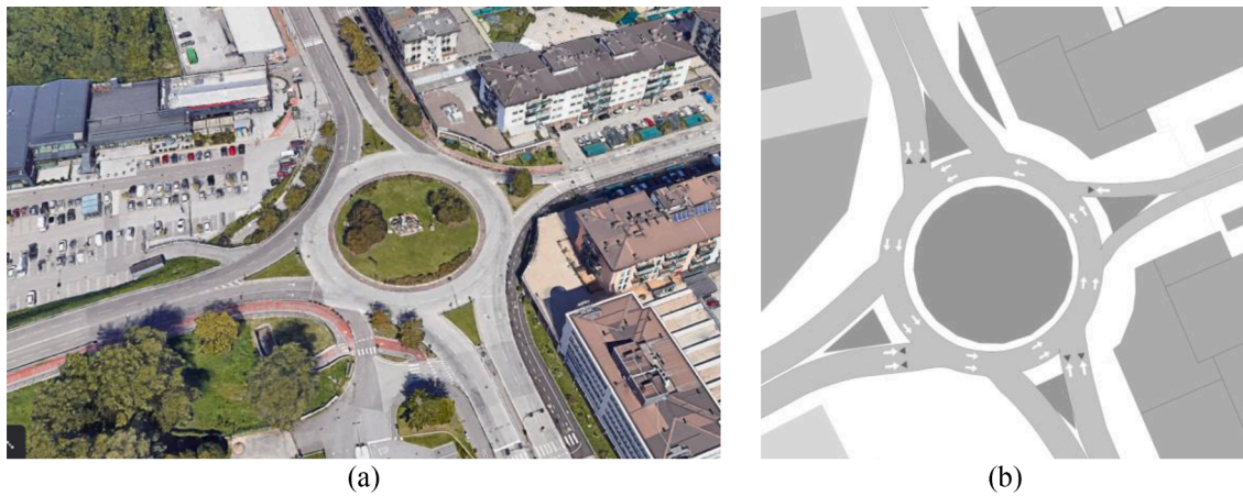
Fig. 2. (a) Example roundabout in Trento, Italy. (b) the roundabout network model built in Aimsun.
