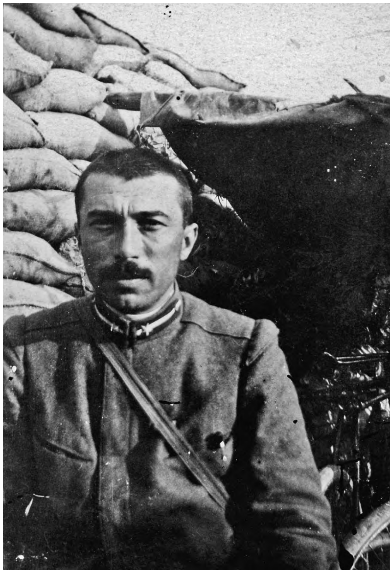
Fig. 18 - Boato in trincea
