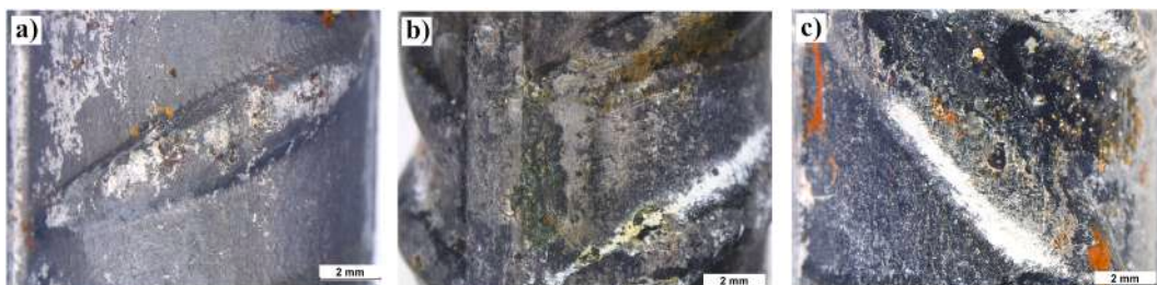
Fig. 8. Images of rebar samples after the CPP in different cement mixtures. PTL (a), PTLCSA (b), Type III-B (c).
