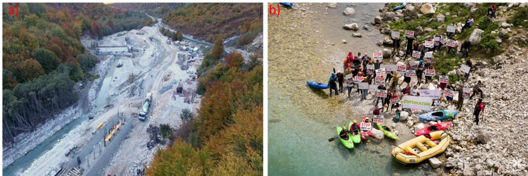
Figure 1. 8. Run off river hydro power plant in Valbona River (tributary of Drin River) in Albania. Valbona valley is a National Park. (a) construction phase in 2018 of hydropower plants in Valbona valley. (b) people from NGO that protest against hydropower plants that are being built in the same national Park (2022).
