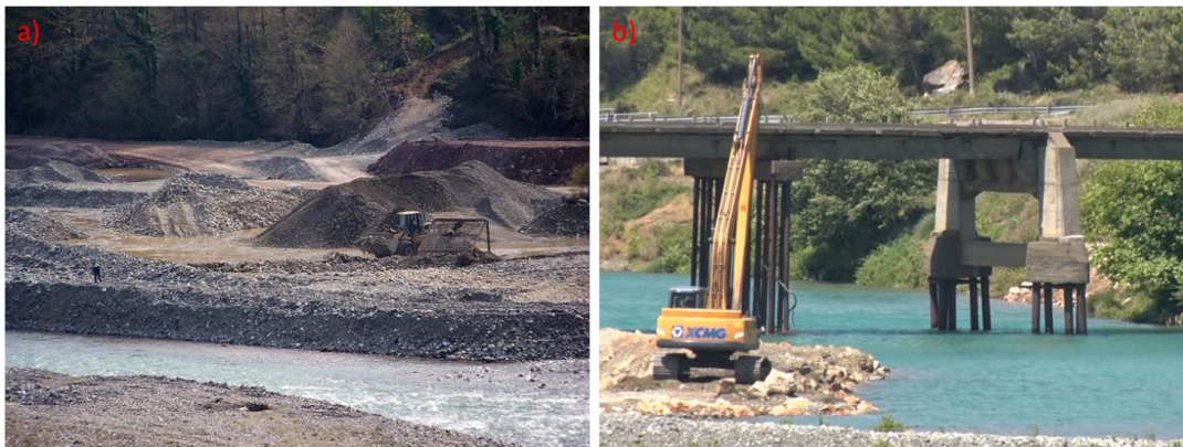
Figure 1. 5. (a) Sediment mining in Shkumbin river. (b) Exposure of the “Bridge Zogu” foundation in Mat River associated with channel incision.
