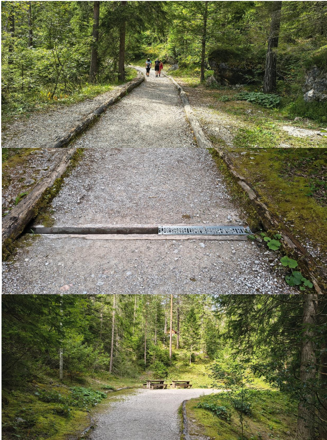
Fig. 1 Example of compacted ground, a drainage channel, and a rest area along a path designated as accessible by the Dolomiti UNESCO Foundation.
