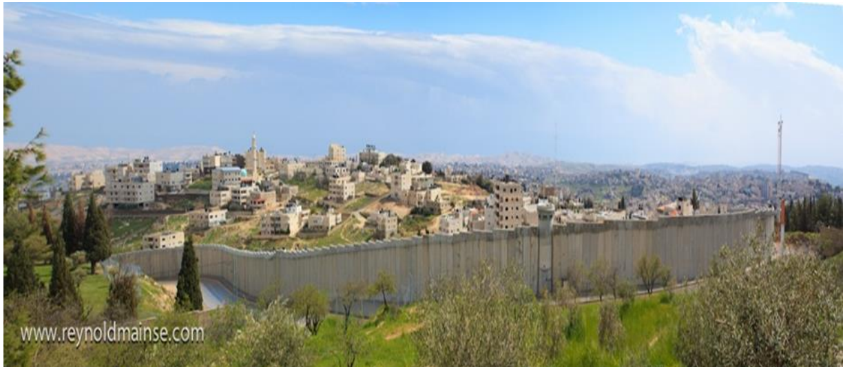
Figure 18: The Wall to the north of al-'Eizariyah where it cuts the bypass road I used to take to Jerusalem through the Mount of Olive. Source: www.reynoldmainse.com
