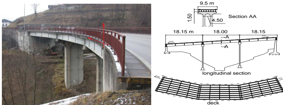
Fig. 2.3 (a) Overview of the SP83 Bridge on the Nogarè River; (b) Plan view, elevation and cross-section of the deck
