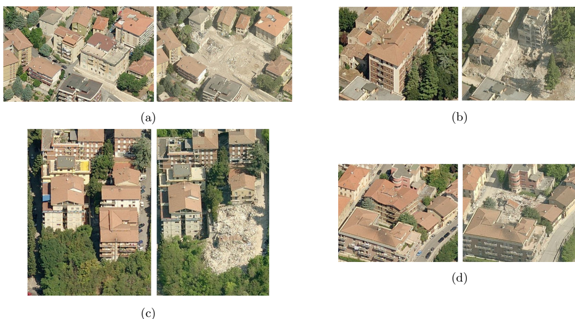
Figure 4.7: (a)-(d) Zoom of the 6 buildings destroyed and correctly detected by the proposed method (Bing Maps, Microsoft Corporation). See Fig. 4.6f for the correspondence of the buildings on the map. As one can notice building was totally demolished after the earthquake.
