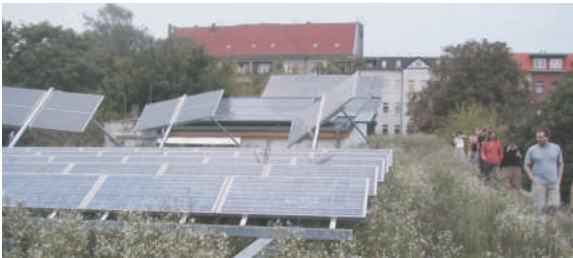
Pannelli solari e tetti verdi, Berlino, Germania Solar panels combined with green roofs, Berlin, Germany
