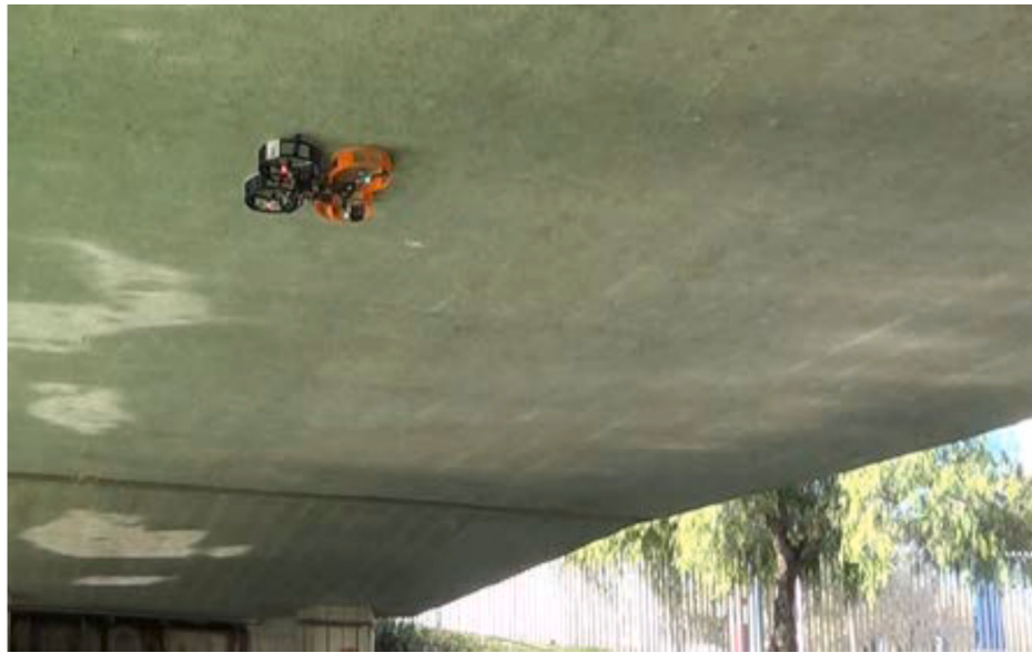
Fig. 9. Drone hovering attached to bridge intrados [114].
