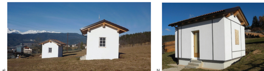
FIG. 10 Test cell A, in the background, and test cell B before retrofit (a); test cell A after retrofit (b).
