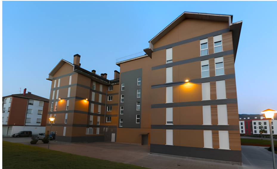
Fig. 6. Selected building photo.
