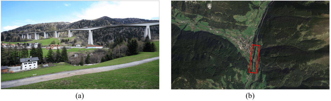
Figure 7.17: (a) Picture of the A22 Colle Isarco Viaduct; (b) Top view of the case-study area, with the viaduct marked with a red rectangle.
