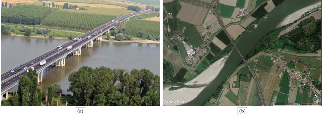
Figure 7.5: (a) Picture of the A22 Po River Bridge; (b) Top view of the case-study area.
