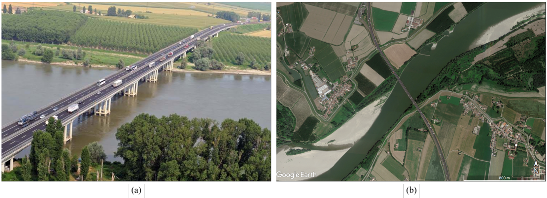
Figure 6.1: (a) Picture of the A22 Po River Bridge, Italy; (b) Top view of the case-study area.
