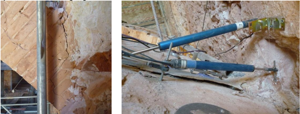
Fig. 5.48 Crack opening in hinges A and CFRP debonding on anchorage
