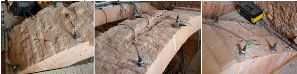
Fig. 5.78 Accelerometers location in the UR vault
