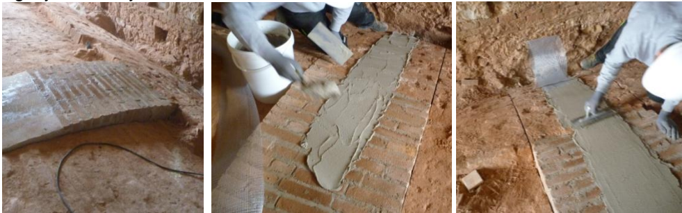
Fig. 5.12 SRG installation, from the left: wetting, first layer and fibres inclusion
