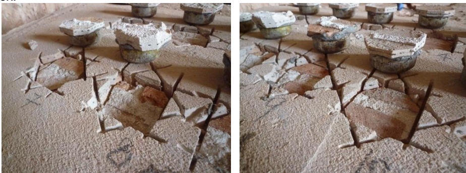
Fig. 5.28 Pull-off tests on SRG with A failure (left) and B failure (right)
