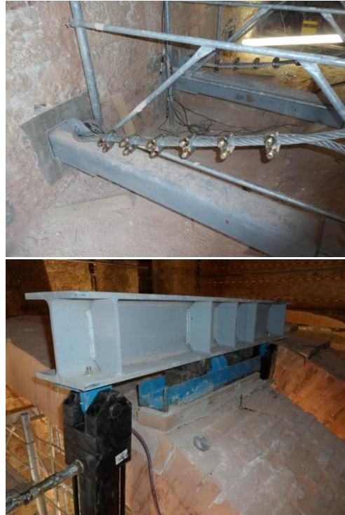
Fig. 5.3 Drawing of the setup (left) Detail on cable link with steel pipe and wall (above) system of load application (below)
