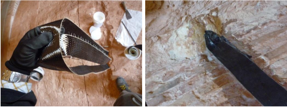
Fig. 5.14 Details of the CFRP anchorage
