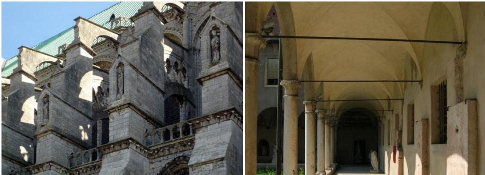
Fig. 2.63 Buttresses in Chartres (FR) (left) ties in S.Fermo's Cloister (right)
