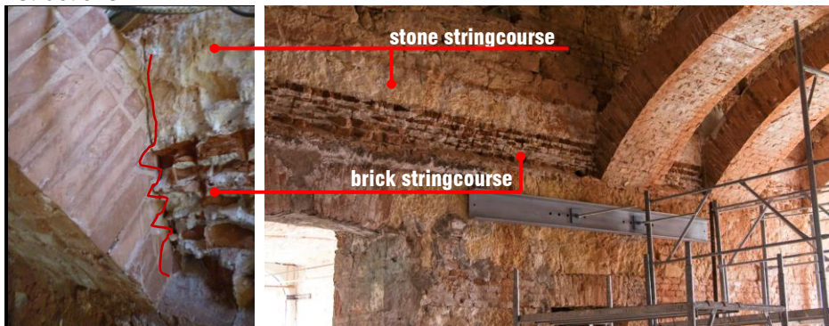
Fig. 5.36 Detail of the stereotomy in supports
