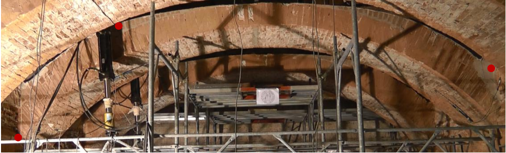
Fig. 5.66 BTRM vault at the maximum displacement
