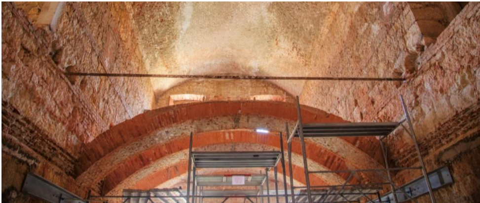
Fig. 5.1 View of the tested vaults inside the castle.
