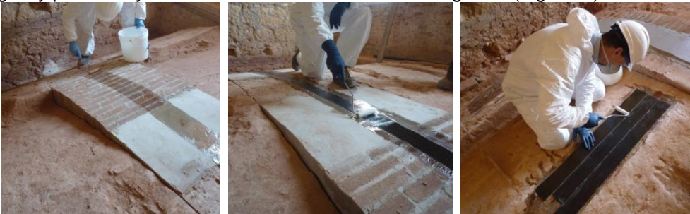
Fig. 5.11 Primer application (left), fibre installation on matrix (centre, right)
