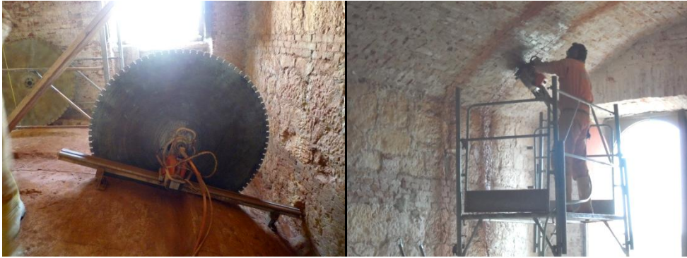
Fig. 5.7 Circular saw (left) and manual finishing (right)
