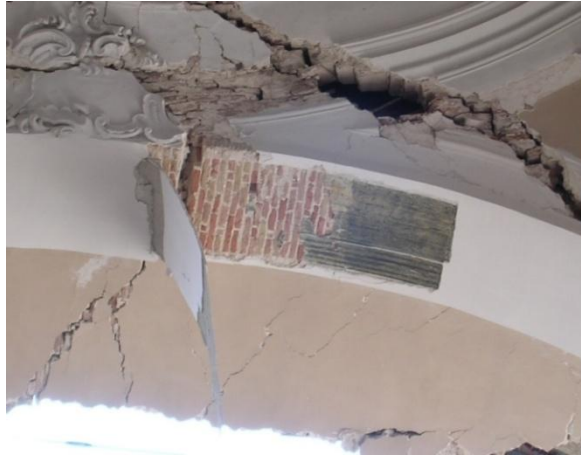
Fig. 2.54 Carbon fibre detachment after the opening of a hinge in the arch (L'Aquila)
