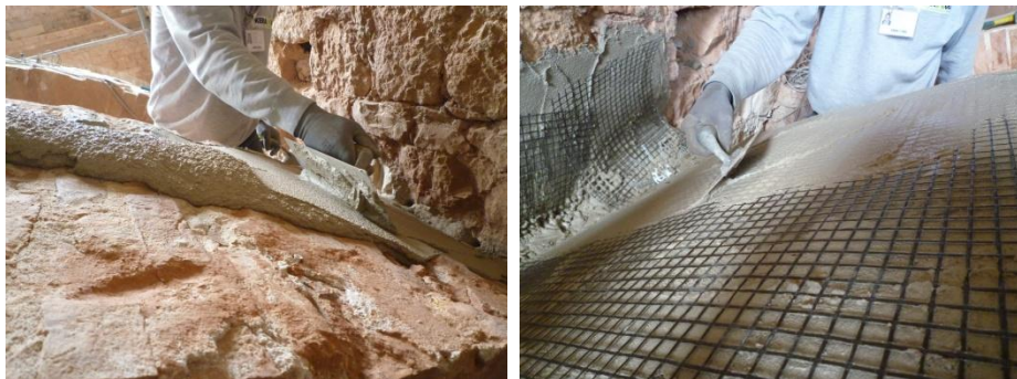
Fig. 5.13 Application of Basalt textile reinforcement with mortar
