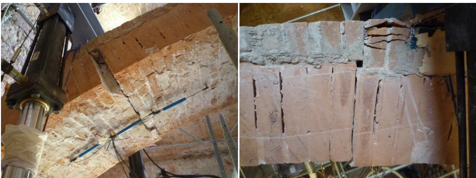
Fig. 5.49 Hinges B, sliding and loss of material (left) and masonry crushing (right)
