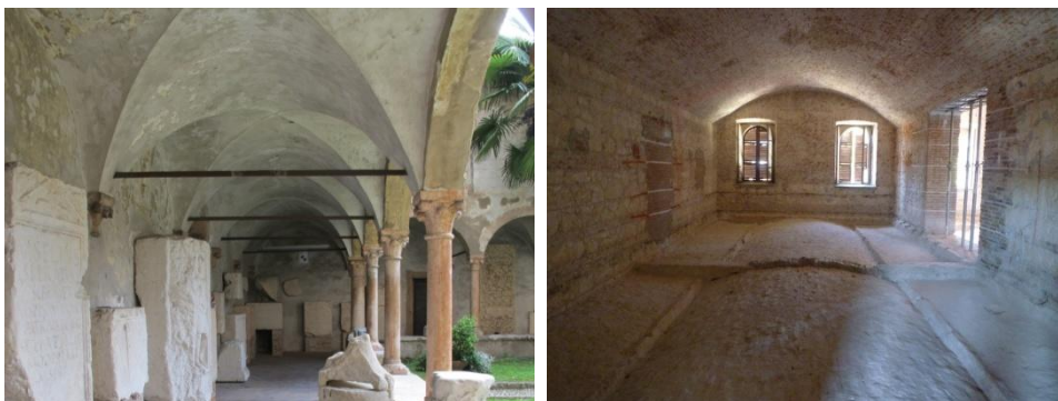
Fig. 2.35, groin vaults of the museum cloister (left), barrel vaults in St. Peter Castle (right)
