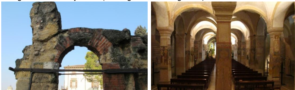
Fig. 2.34 Arch in the Roman Theatre (left), groin vaults in S. Fermo's lower church (right)
