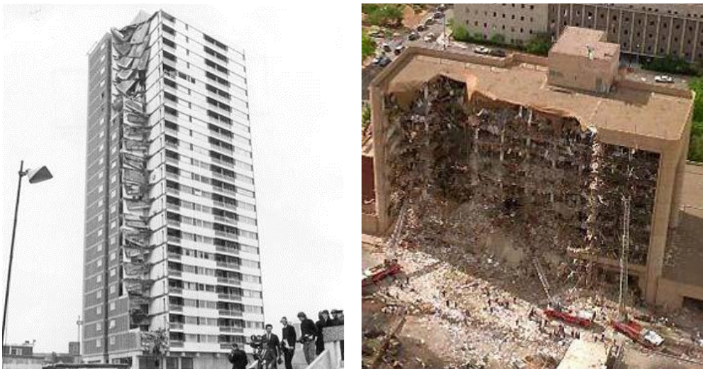
Figure 2.1 - Ronan Point Building and Alfred P. Murrah Building collapses
