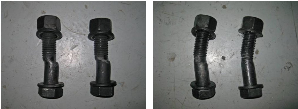
Figure 4.16 - Bolts deformation at collapse
