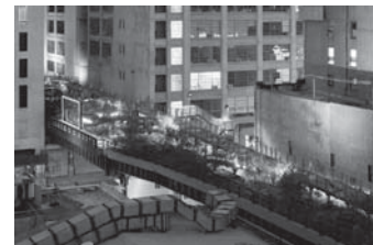
The High Line New York, 2011 (in progress)
