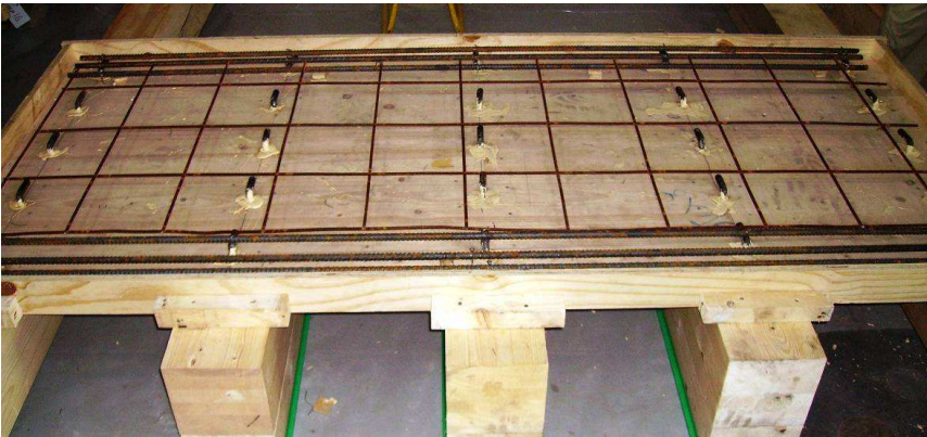
Fig. 87 Specimen view in the reinforced laying phase
