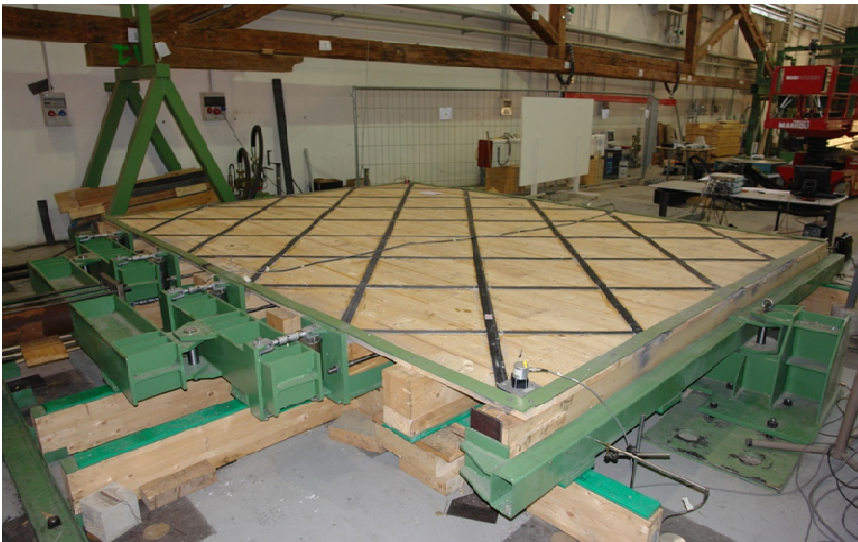
Fig. 67 Floor reinforced with FRP strips
