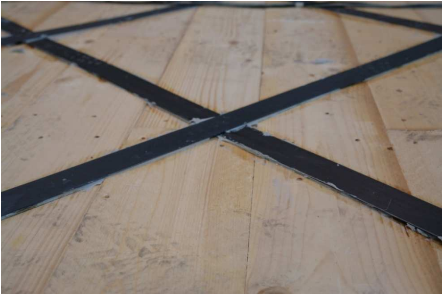
Fig. 69 Detail of connection FRP strips-simple layer
