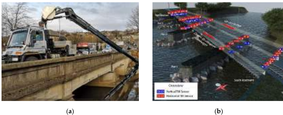
Figure 2. (a) BridgeCat technology for bridge inspection [40]; (b) Layout of the Structural Health Monitoring (SHM) system installed at the Lamington viaduct (courtesy of Network Rail).
