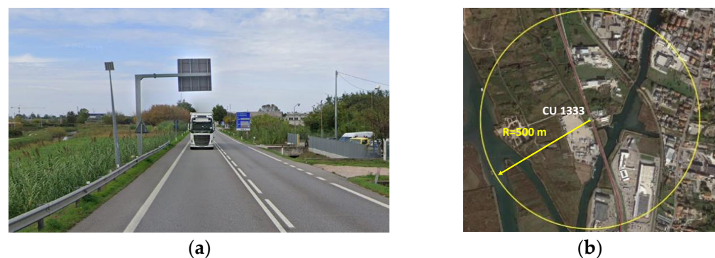
Figure 4. Control unit 1333 on the national road n.309: (a) installation site with two lanes; (b) surrounding 500 m radius area (Google Earth).
