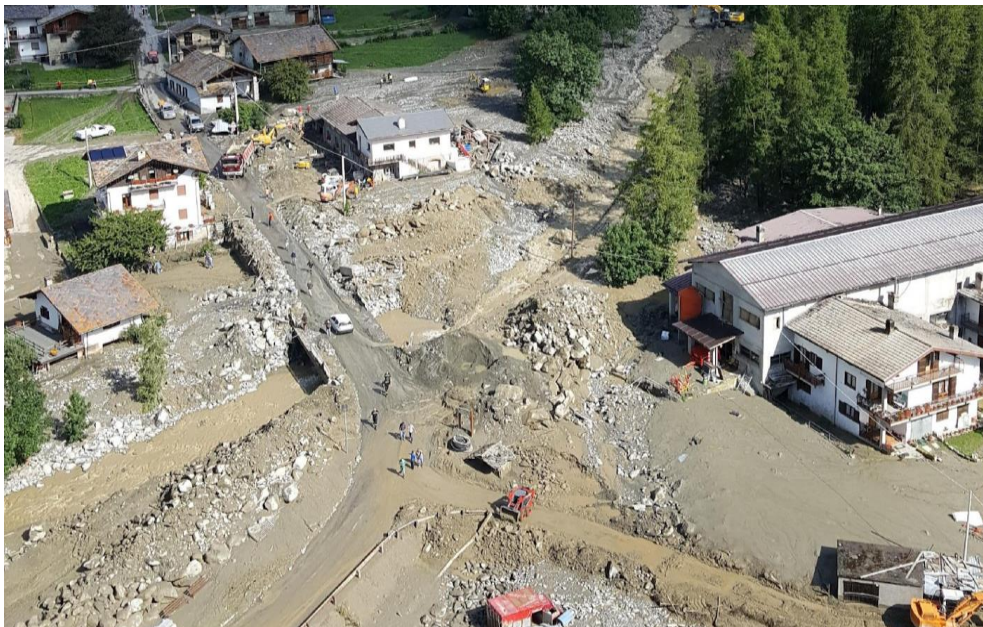
Figure 1. Consequences of a bridge clogging in the village of Voueces, Ollomont municipality (AO), following the debris flow event of August 2017.
