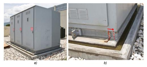
Fig. 2.5 a) Metal-enclosed load interrupter switchgear (MELIS) equipment at the U.S. Embassy. b) and displacement due to the 2010 Haitian quake (PGA=0.16g). (From Goodno et al., 2011).
