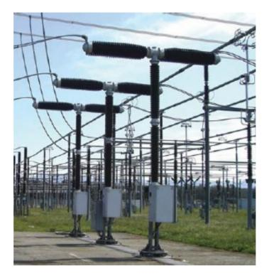
Fig. 2.32 Installation of the seismic isolation system with Wire-Rope devices at the base of a HV circuit breakers in a power plant (from Alessandri et al., 2014).
