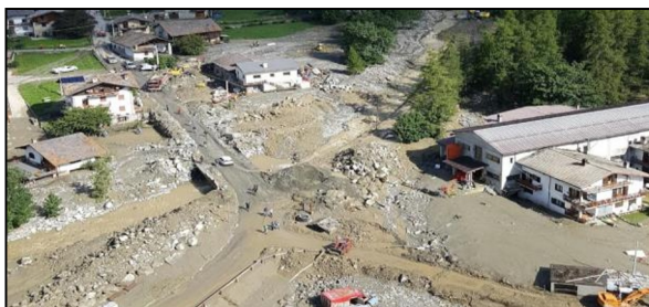
Fig. 1. Consequences of a bridge clogging in the village of Voueces, Ollomont municipality (AO, Italy), following the debris flow event of August 2017.
