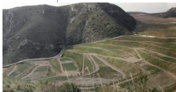
The rehabilitation of Garraf's dumping area, Barcelona, Battle, Roig and Gali.
