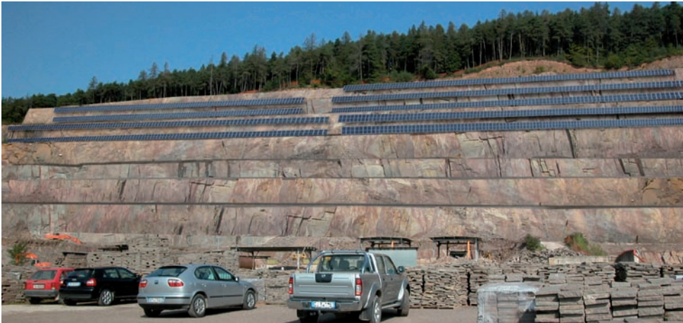
Fornace: photovoltaic system in the upper desused steps contemporary with the quarrying as per 2004 plan.
