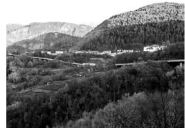
New mobility infrastructure in the Cembra valley, 2009.
