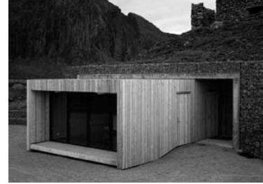
Snohetta AS, Tourist route Ev10, Rest area, parking and toilet facilities, 2007.
