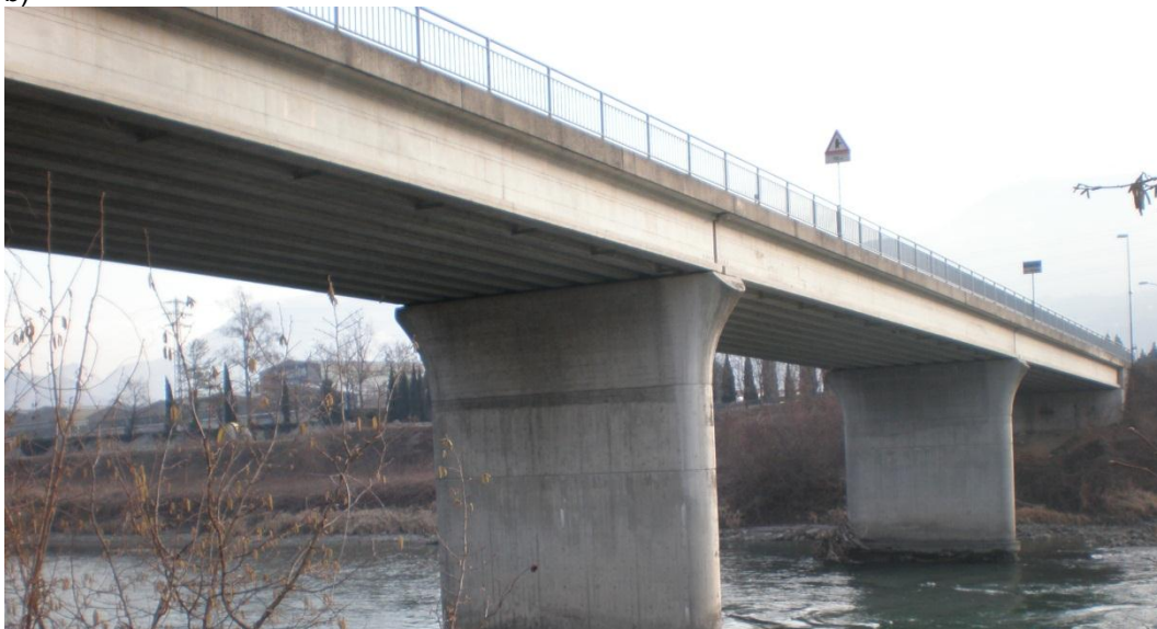
Fig. 25: a) and b): “Adige Bridge”, Municipality of Rovereto (TN, Italy)
