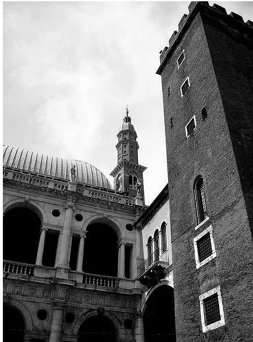
Figure 6 Tormento tower in Vicenza: thermal load crack
