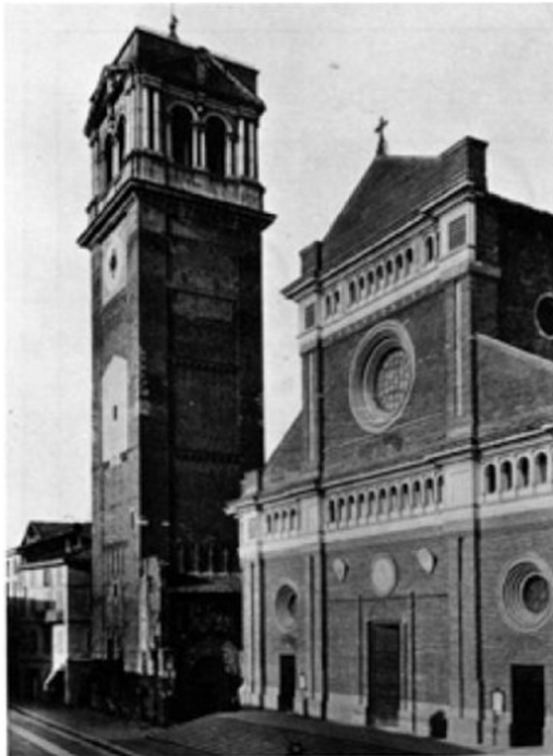
Figure 7 Pavia civic tower before collapse
