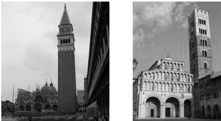
Figure 2, 3 Examples of isolated tower (San Marco bell tower) and connected to other buildings (Bell tower in Lucca)
