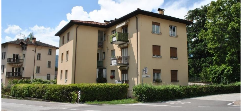
Figure 4.10 - From top to bottom: view of the residential building in Povo, survey campaign with LIDAR sensor, total station, MMS and telescopic pole. Images by LA-MARC.
