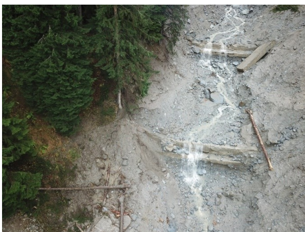
Fig. 1. Remnants of two destroyed check dams along the Rio Rotiano.
