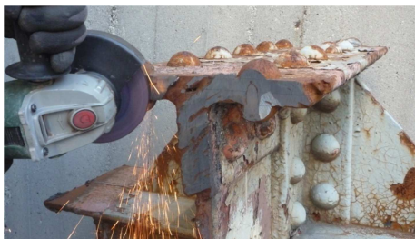
Figure 178. Surface treatment.
