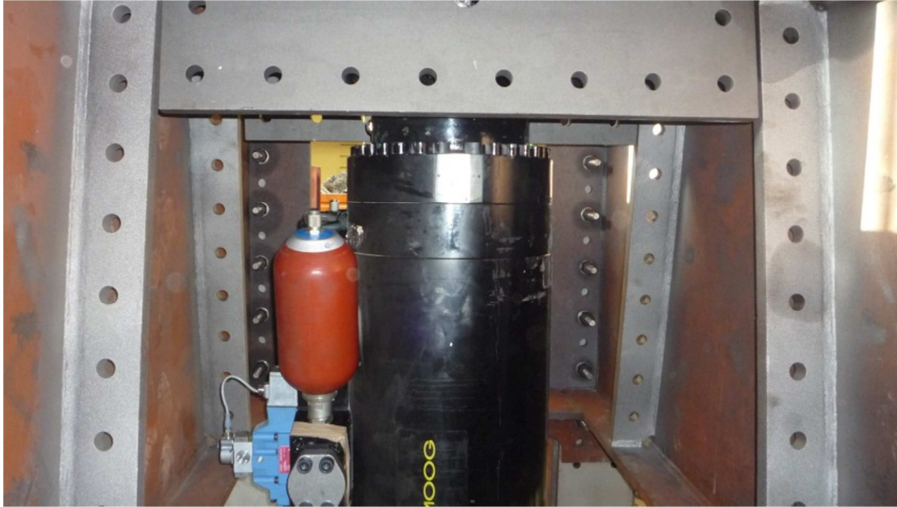
Figure 301. Bolted joints during the assembly phases.
