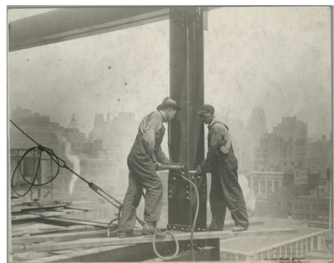
Figure 12 Rivet installation.
