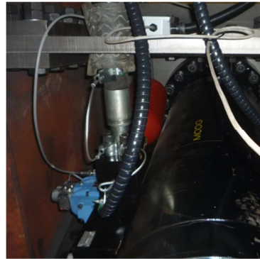
8. Oil and data cables.
