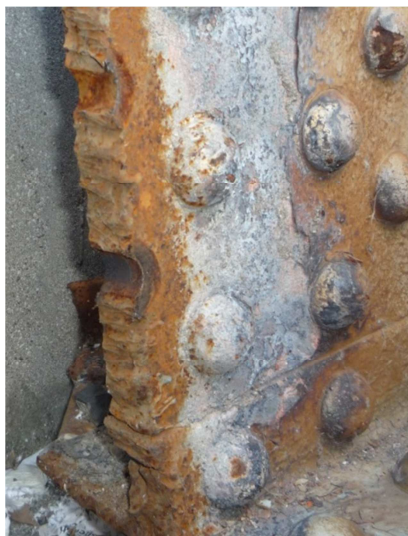
Figure 184. Rivets hole (Girder "B").
