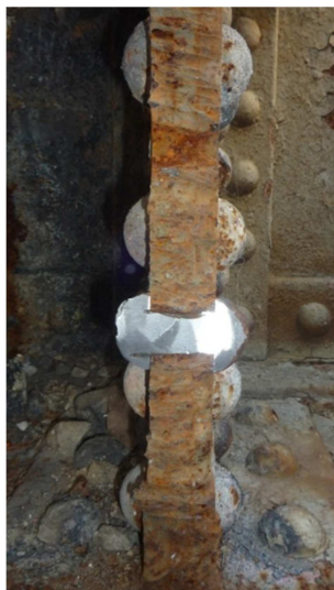
Figure 183. Rivet section (Girder "B").
