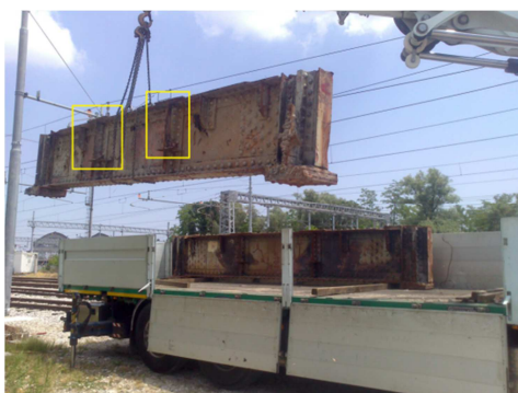
Figure 58. Cross girders and longitudinal intersections.
