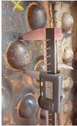
Figure 186. Diameter and shank gauge.
