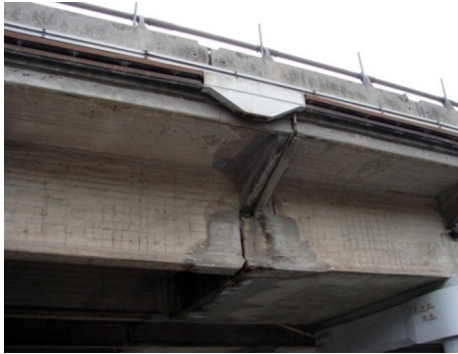
Figure 3.3: Detail of one Gerber saddle
