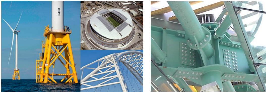
(a) Traditional hollow section joints and the applications
